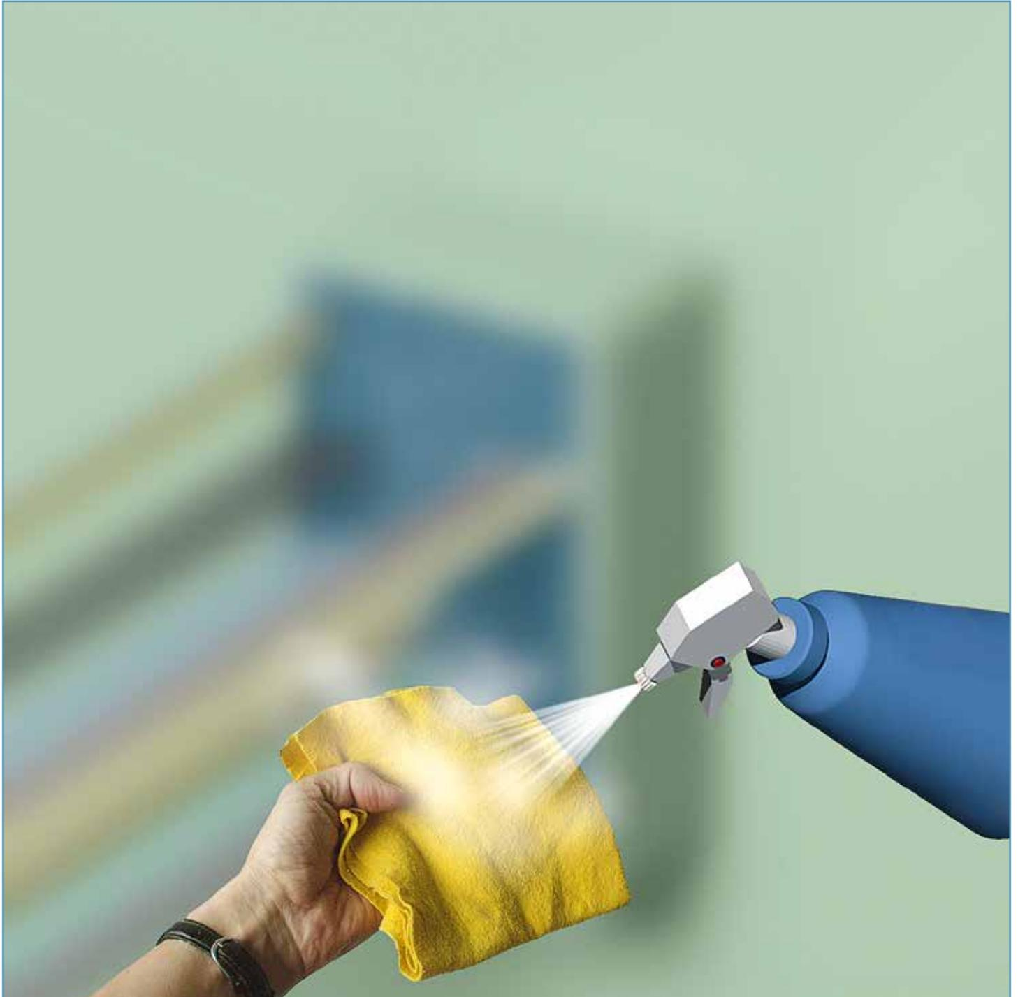
To smooth the surface of the NOFIRNO® sealant layer, a cloth is sprayed with water. This prevents the sealant from sticking to the cloth.
