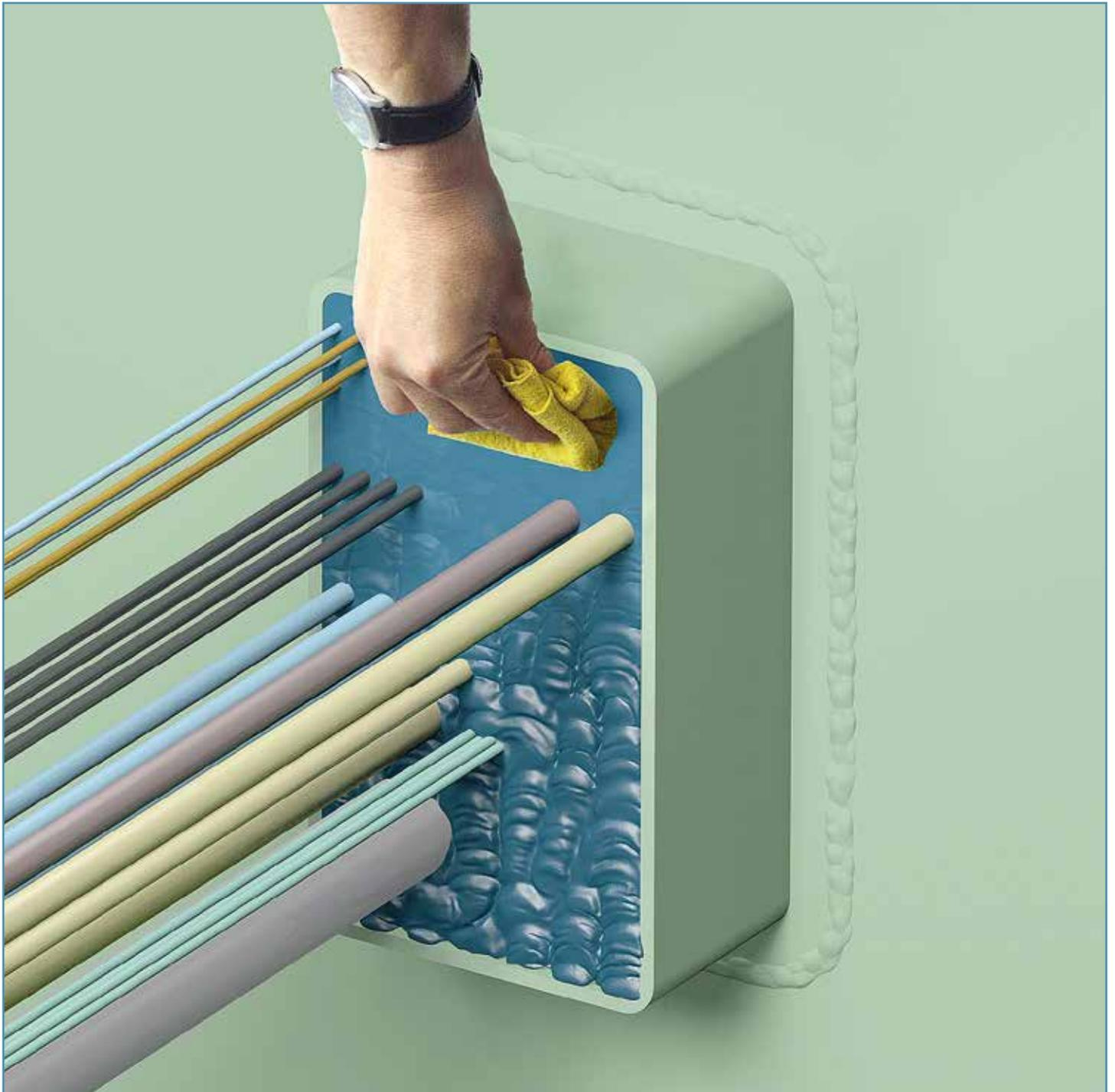
The cloth is then used to press down the sealant layer flush with the end of the transit frame.
