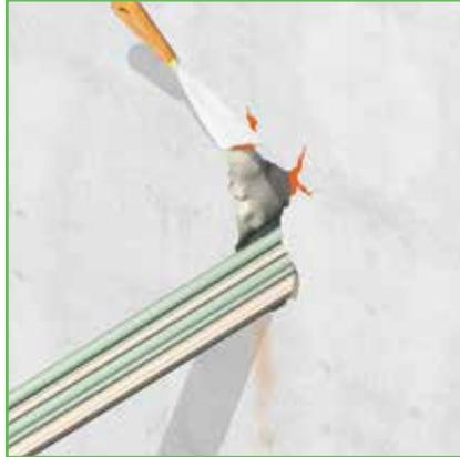
2) If there are large irregularities in the wall around the opening, they should be locally smoothed with DRIFIL® or NOFIRNO® sealant. NOFIRNO® sealant has highest mechanical properties.
