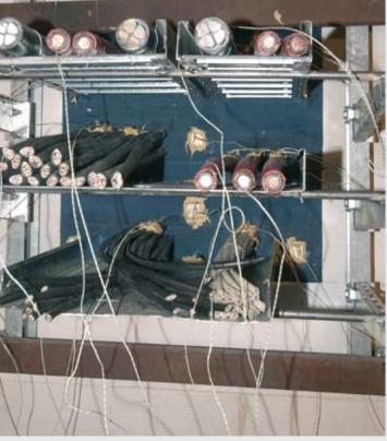
1) ACTIFOAM<sup>®</sup> rubber sheets are cut into strips fitting to the size of the walls inside the conduit opening. For this purpose ACTIFOAM<sup>®</sup> sheets with a thickness of 25 mm are used. Fitting sheets are placed underneath the busbar casing.
