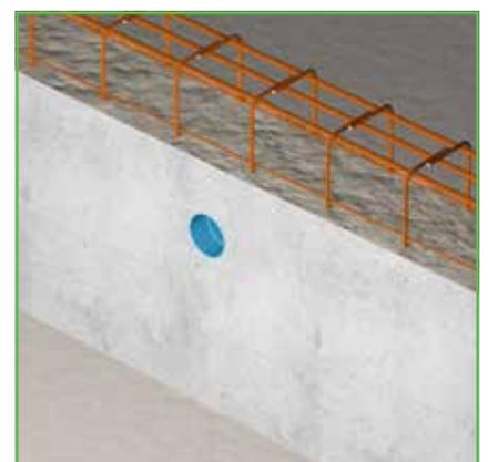
9) The CSD® fixation pieces that are affixed to the formwork can be re-used for subsequent projects.
