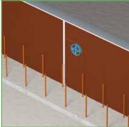
1) After marking off on the formwork, CSD® fixation pieces suitable for CSD® conduit inlets are fastened by means of nails or screws.
